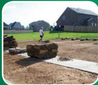
Photo credit: Barry Tinning, Tetra Tech
