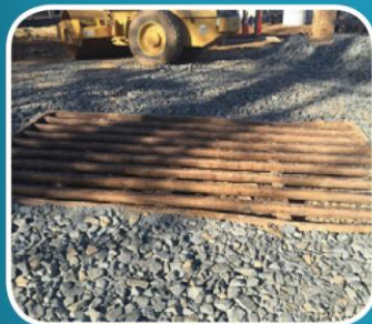
Rumble pad construction exit.
